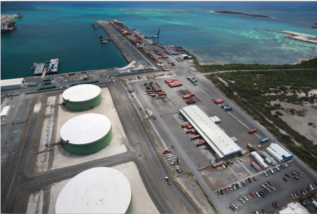
Before (Old Terminal)
