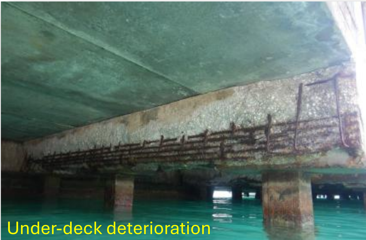
Under-deck deterioration
