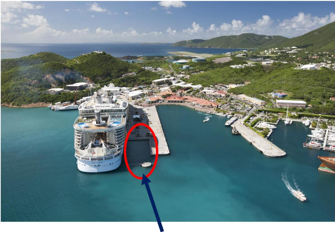
The notch at the end of the cruise ship pier at the Austin Babe Monsanto Marine Terminal in Crown Bay, St. Thomas will be filled in to provide more stability for the ships berthed at the pier and less damage to the pier.
