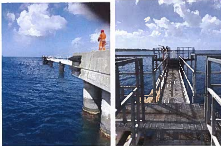
The catwalk at the pier in Frederiksted has been repaired post-storms.
