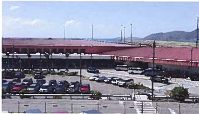
The entire roof of the CEKA Terminal will be replaced. Expected completion – November 2018.
