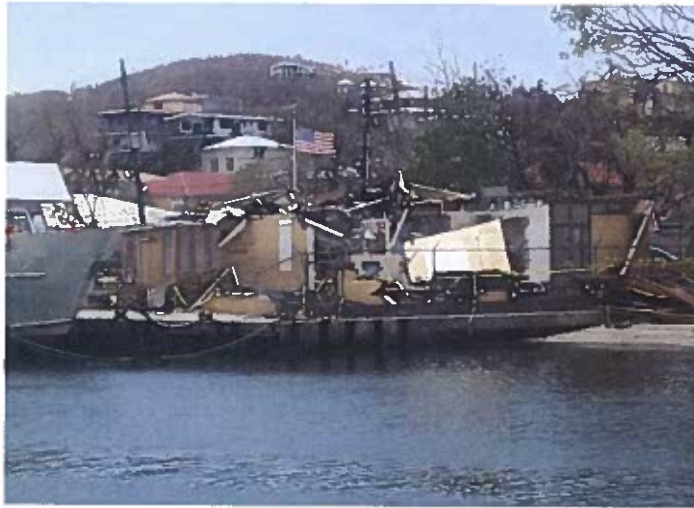
Damaged US Customs Building in Cruz Bay
